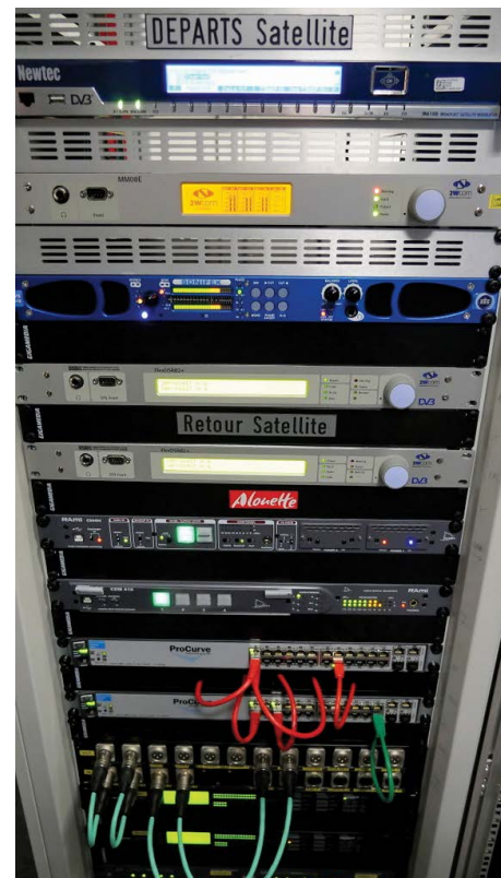
Satellite distribution equipment shown in Alouette's rackroom: uplink encoders and confidence receivers.
